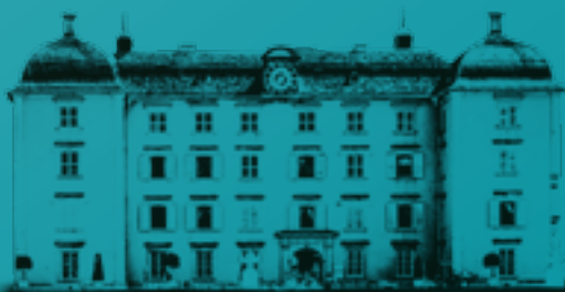
SCHWETZINGEN SOU AG | Headquarter
